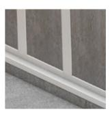
Connection joints between precast concrete elements need to be sealed after installation of the individual segments. In addition, all transitions/connections to in situ concrete must be sealed – typically using the Sikadur®-Combiflex® SG System.
